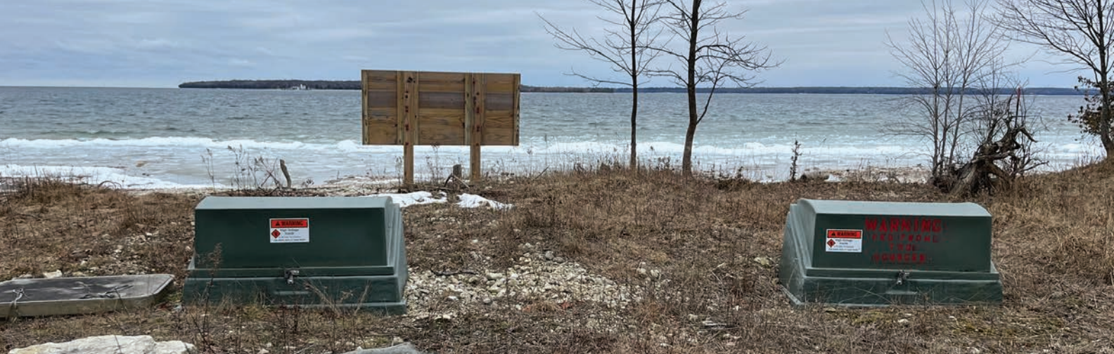
SECTIONALIZING CABINET WITH NEW CABLE
