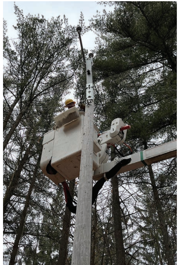
Above: Mike and Mitch (from Karcz) trimming pines from the lines. Right: Mike installs a pole extension to replace a broken pole top on Detroit Harbor Road.
