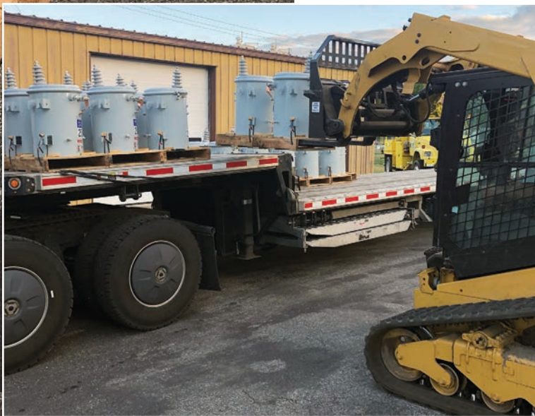
Unloading the new 25KVA transformers was much easier with the skidsteer and the forks.
