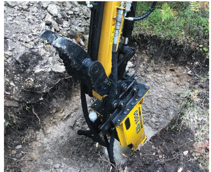
Breaking through solid limestone in order to set a pole.
