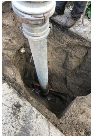
Top row, left to right: Vacuum excavator begins opening the trench after the blacktop was removed. Conduit and duct safely located. Fiber duct cleaned and recoupled. Right: Filling the trench with gravel. Below right: Fiber being fed into the now cleared duct.
