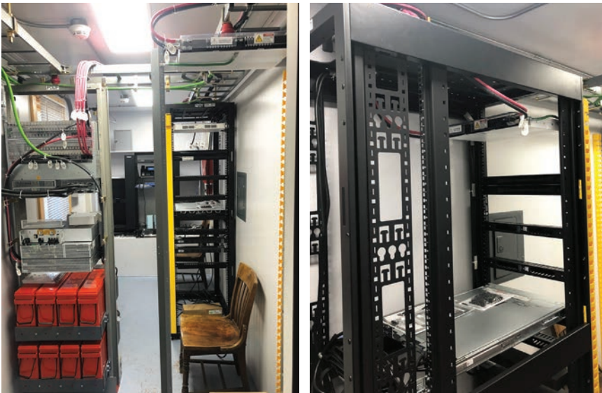
DC Power Supply and racking awaiting equipment being shipped from NRTC.
