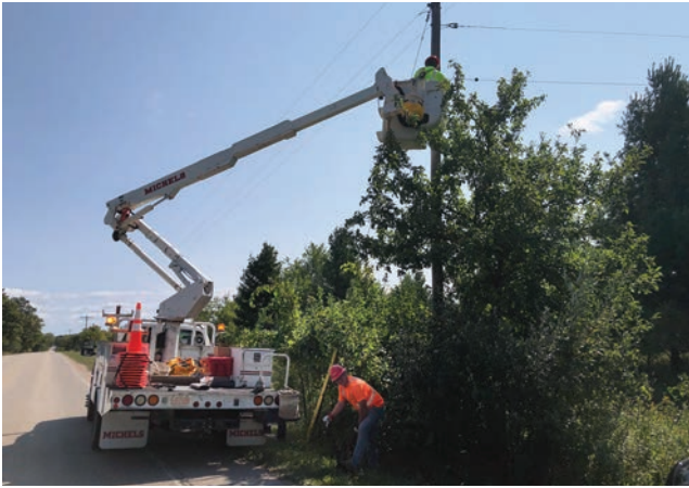
Left: Michels crews framing poles to pull up the strand. Above: Michels, Quantum, and cooperative crews.
