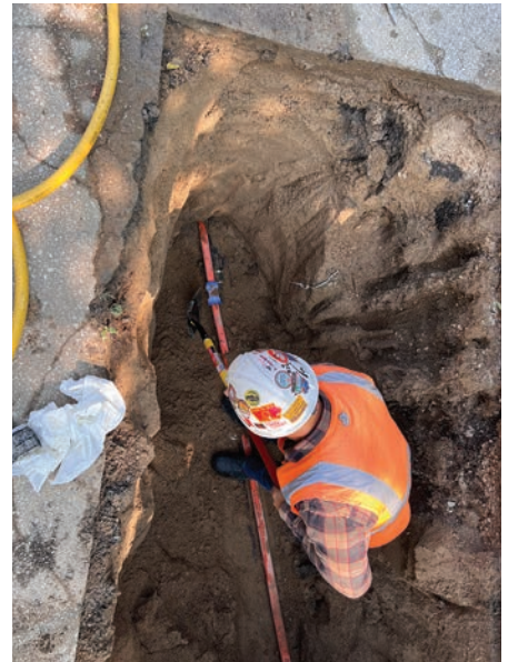
Top row, left to right: Vacuum excavator begins opening the trench after the blacktop was removed. Conduit and duct safely located. Fiber duct cleaned and recoupled. Right: Filling the trench with gravel. Below right: Fiber being fed into the now cleared duct.
