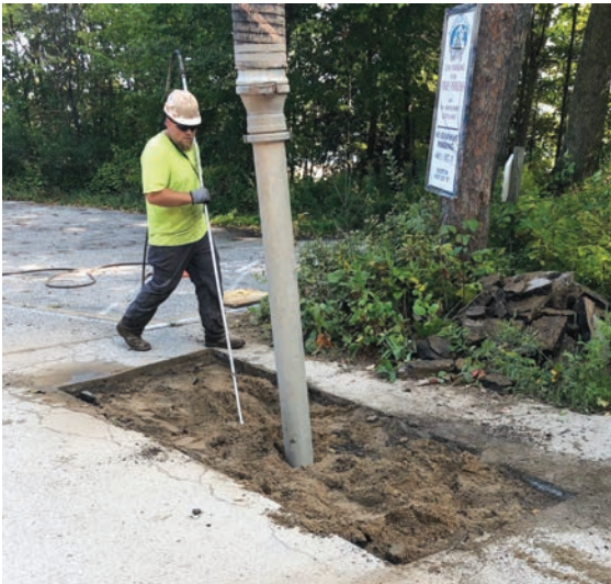
Top row, left to right: Vacuum excavator begins opening the trench after the blacktop was removed. Conduit and duct safely located. Fiber duct cleaned and recoupled. Right: Filling the trench with gravel. Below right: Fiber being fed into the now cleared duct.
