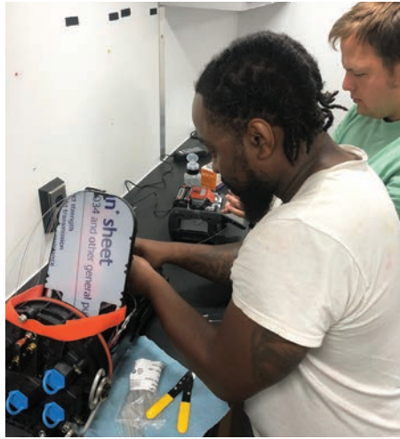
Above left: Clint splicing at the Cellcom tower. Above center: Clint and Walker splicing Nsight Fiber at the cooperative. Above right: Clint preps the trays. Below left: Clint and Kolin splicing Nsight fiber at the cooperative. Below: Kolin, Walker, and Clint prepping WIEC fiber for splicing at the cooperative.
