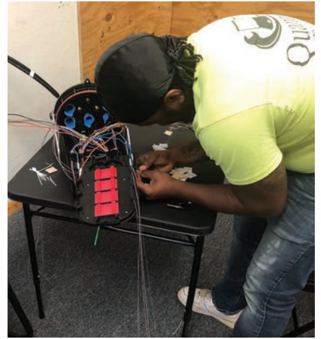
Above left: Clint splicing at the Cellcom tower. Above center: Clint and Walker splicing Nsight Fiber at the cooperative. Above right: Clint preps the trays. Below left: Clint and Kolin splicing Nsight fiber at the cooperative. Below: Kolin, Walker, and Clint prepping WIEC fiber for splicing at the cooperative.
