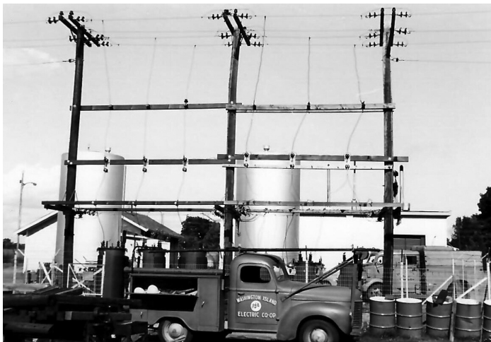
Substation construction showing the International truck (early 1960s).
