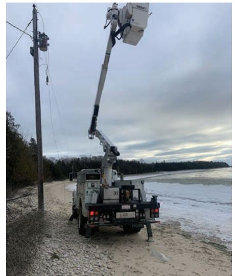
Believe me when I tell you that this is not our idea of a fun day at the beach, but we were lucky the ground was firm enough that we could get the truck to this pole to make repairs.
