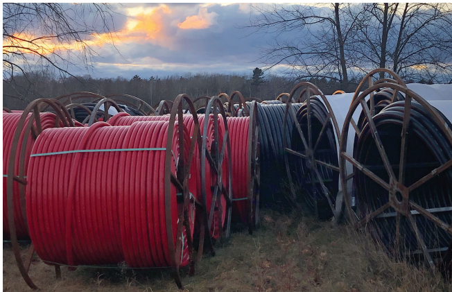
Reels of cable in conduit and fiber duct (left) and system sectionalizing cabinets and fiber hand holes (right) awaiting installation on Lobdell Point Road.
