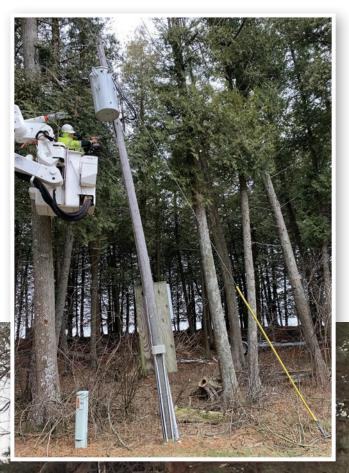
Overview: the large pine that is now under the lines was once across all three phases. Above: While not caused by this current round of storms, this pole was leaning severely and required straightening prior to fiber being attached. Trees going across the lines had actually pulled the guy anchor out and the lines were sagging.
