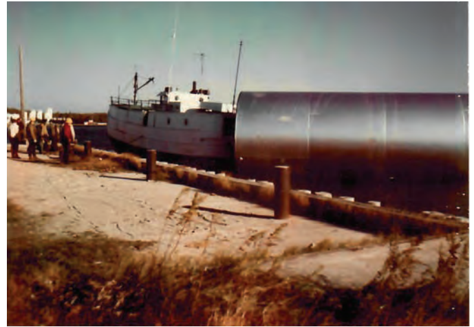
One of the fuel tanks used to store diesel fuel for the engines being delivered by the freighter American Girl . The 10,000-gallon tank was floated to the Island approximately 1959.
