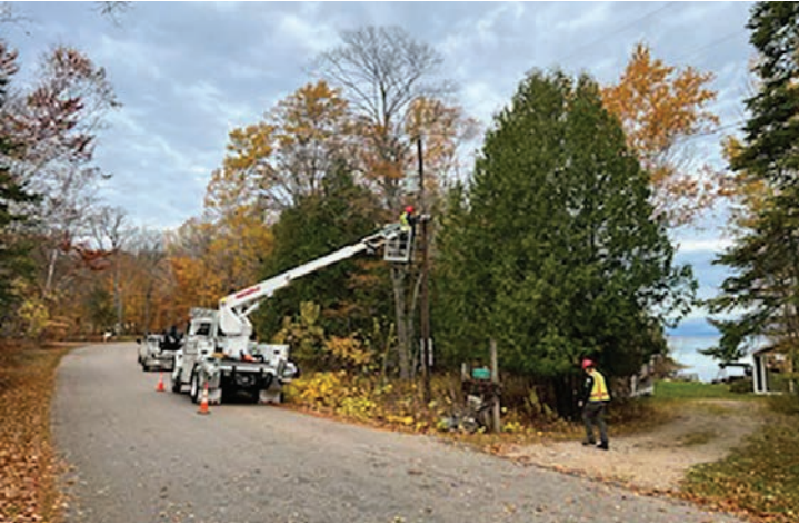
Michels running fiber on Green Bay Road (above) and over-lashing 96 strand fiber on Townline Road (right).
