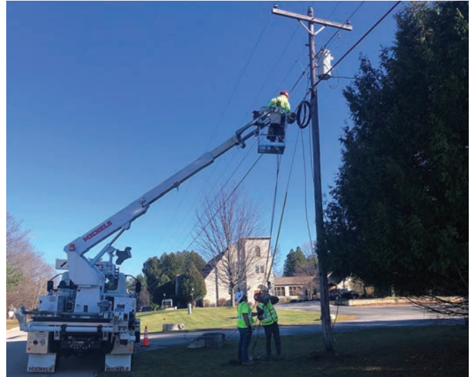
Michels running fiber on Green Bay Road (above) and over-lashing 96 strand fiber on Townline Road (right).
