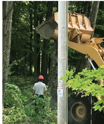
Left: Mike Jorgenson prepares to cut an oak that was threatening three-phase lines running south while John Mann pushes with the loader Right: A dead birch branch that came in contact with the lines and then dropped to the ground started the above fire. Luckily the ground was wet enough that the fire was contained and did not spread.
