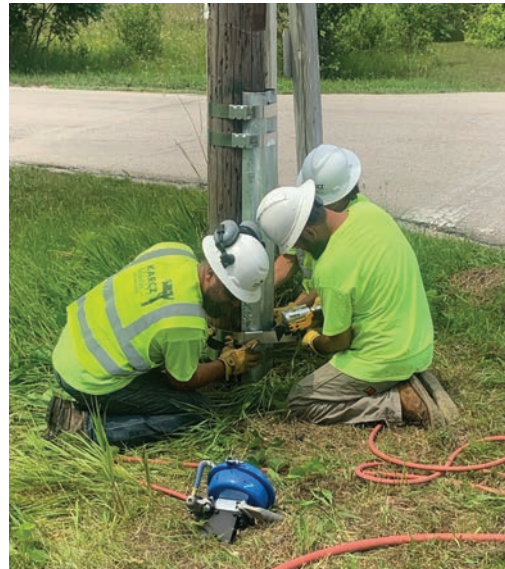
Karcz crew securing the reinforcement/repair to the pole using heavy banding straps. Right: A completed reinforcement/repair including channel, banding and cover.
