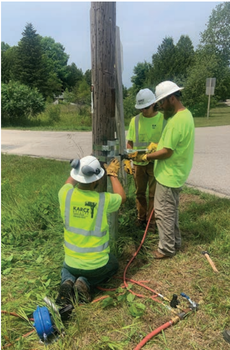
Karcz crew securing the reinforcement/repair to the pole using heavy banding straps. Right: A completed reinforcement/repair including channel, banding and cover.
