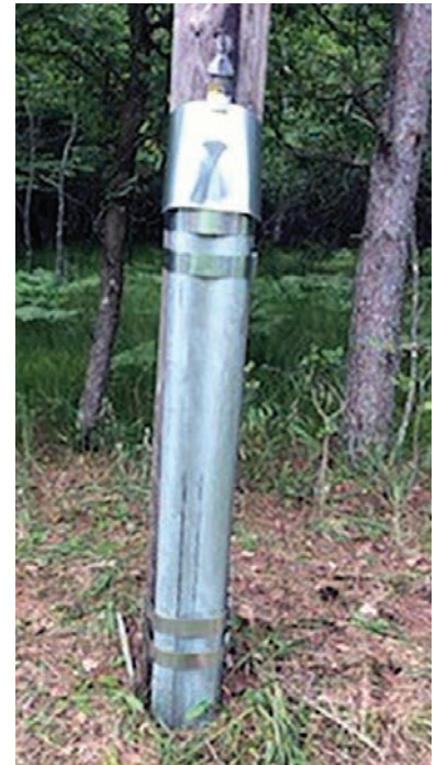
Karcz crew securing the reinforcement/repair to the pole using heavy banding straps. Right: A completed reinforcement/repair including channel, banding and cover.
